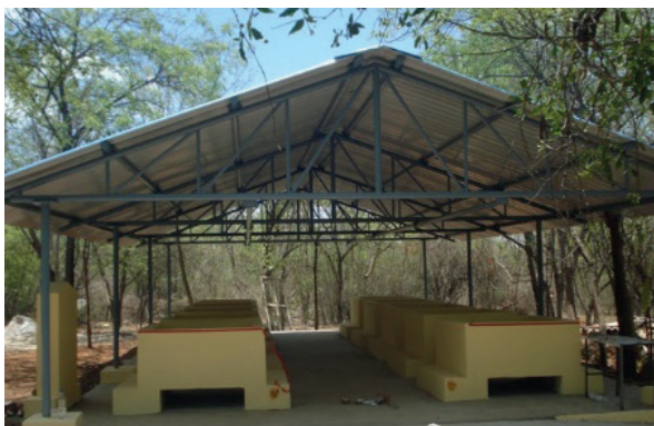
Poultry waste management unit
